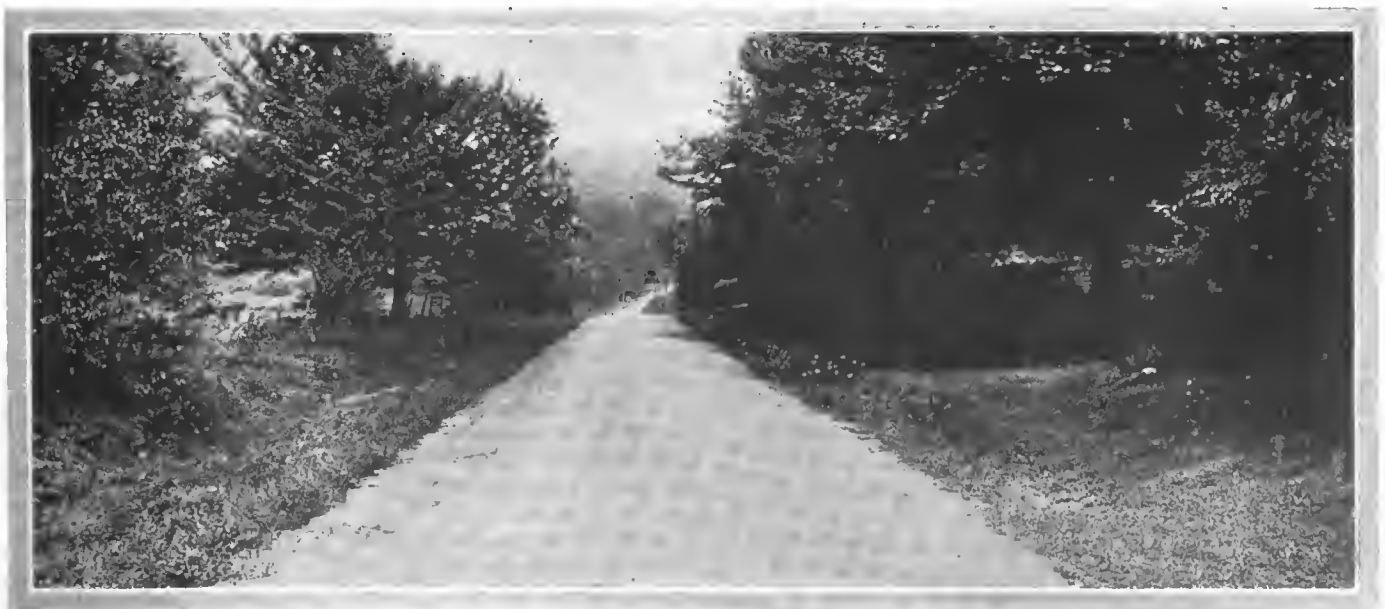
A STRETCH OF PICTURESQUE ROADWAY ON THE MONTGOMERY TURNPIKE AT ROSEMONT, PA., RECENTLY TREATED WITH TARVIA.
